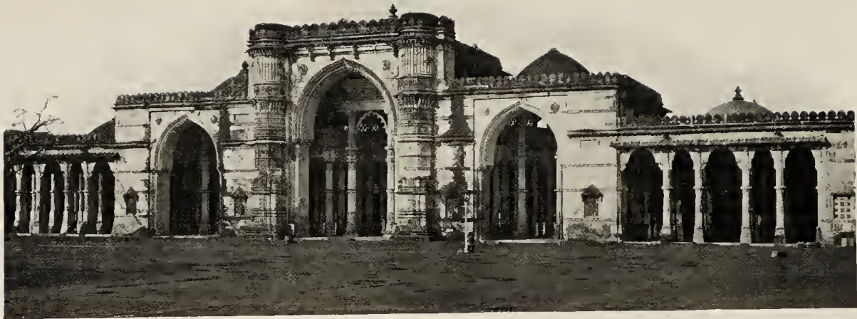
Exterior of Mohammedan Temple at Ahmedabad
